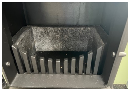
3x bricks with grate upstand in front.
